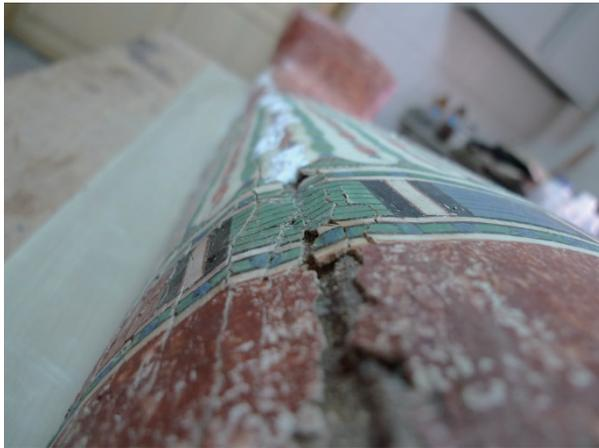
Fig.18 Distorted surface with misaligned break edges
