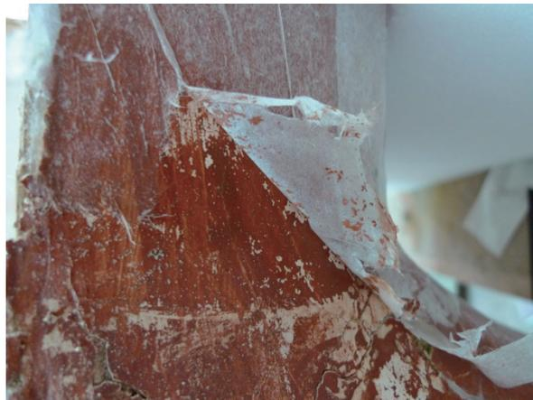
Fig.20 Sections of red paint lifting off with paper facing
